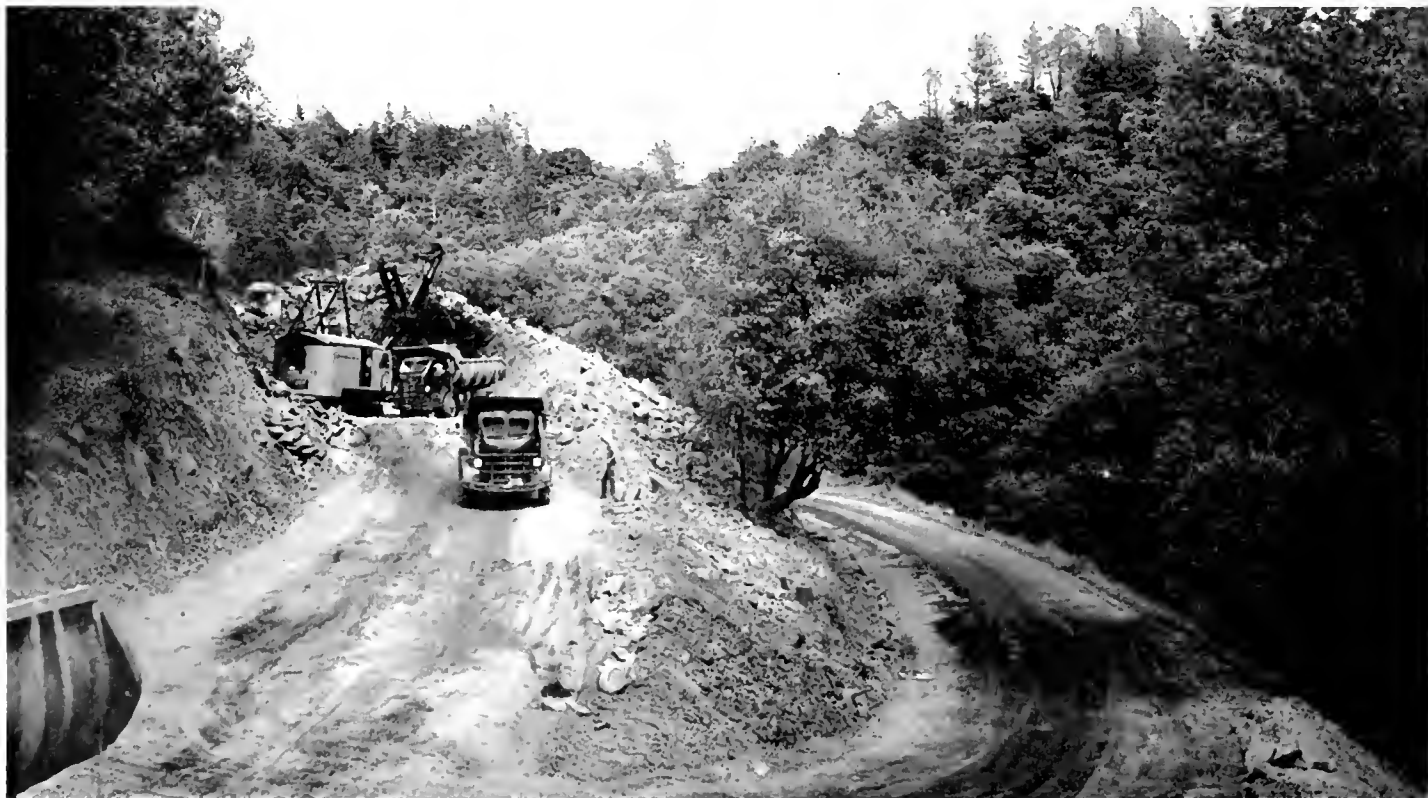
Construction between Jackson and Pine Grove in Amador County
